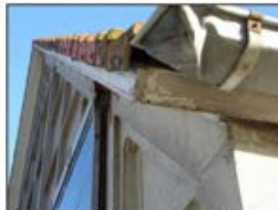
Figuur 12. Opening tot gootbekisting.
